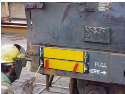
INITIAL PREP FOR DELINEATORS BEING HELD IN PLACE BY MAGNETS.
